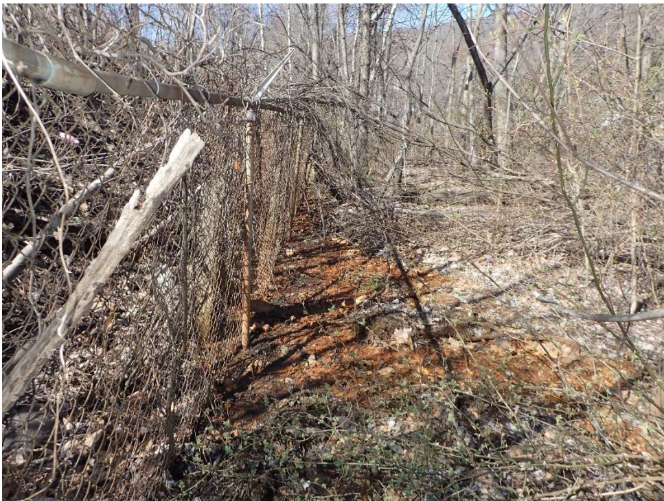
PHOTO 20: Boggy, wet area of possible seepage with rust stains at toe looking southwest.
