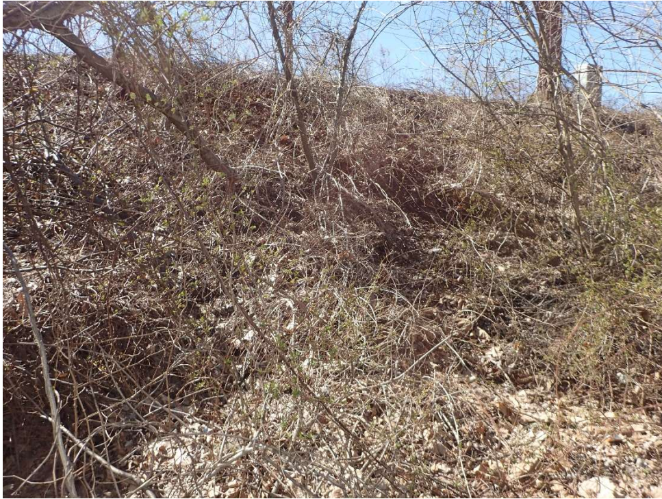
PHOTO 19: Previous topsoil sloughing covered with vegetation growth at downstream embankment looking south.
