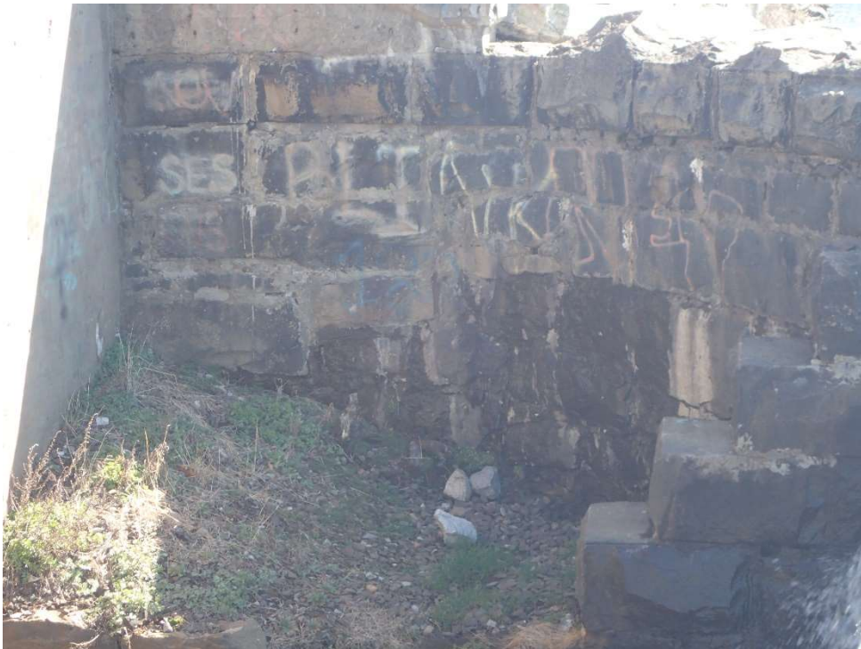
PHOTO 6: Joint deterioration and seepage at eastern spillway wingwall looking northeast.
