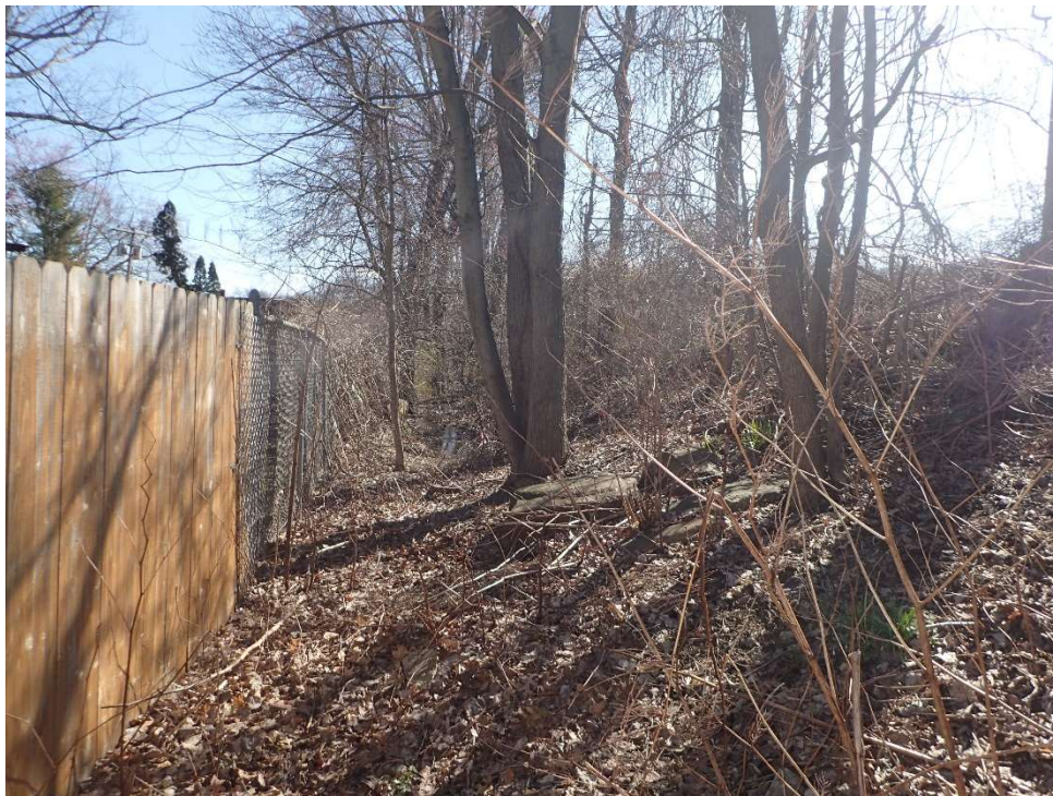
PHOTO 12: Downstream embankment with full-grown trees looking northeast.
