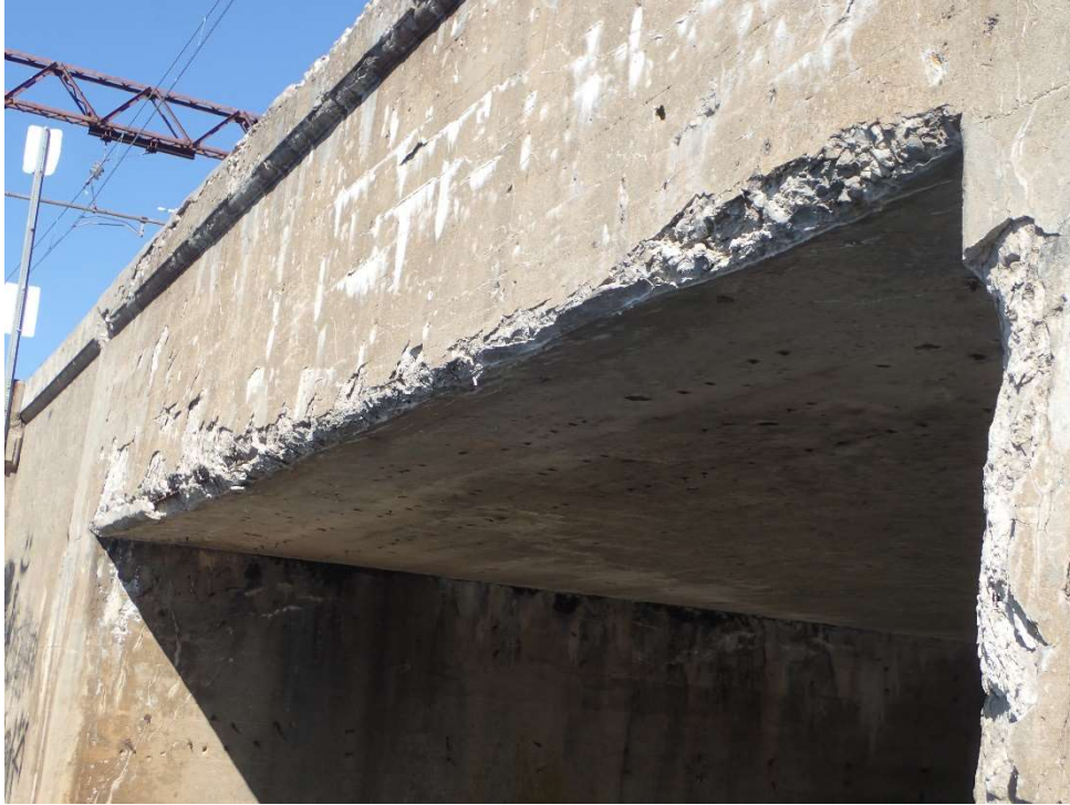
PHOTO 5: Close up of upstream bridge deterioration with spalls and exposed reinforcement looking northwest.
