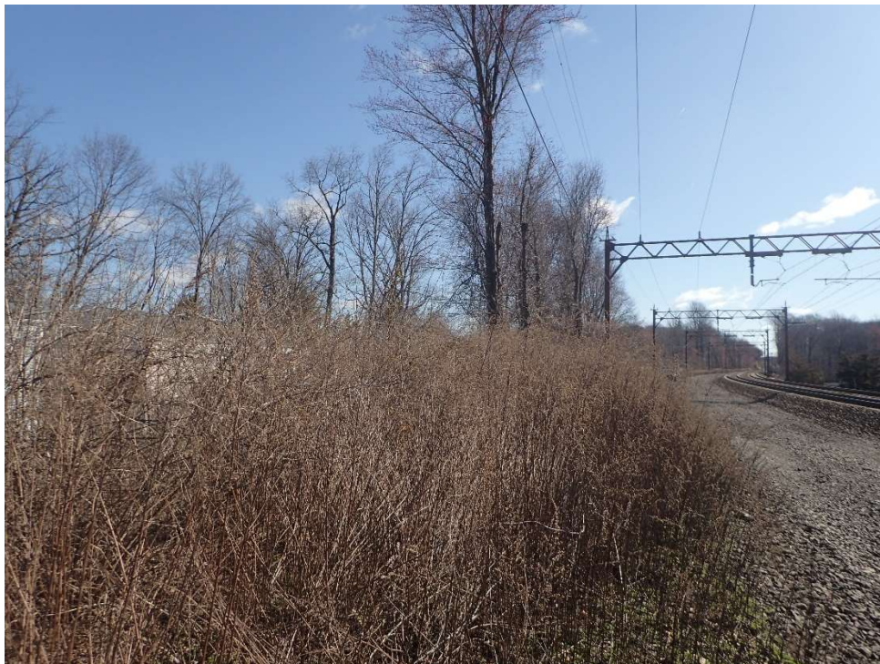
PHOTO 14: Previous area of clearing with excessive vegetation growth along downstream embankment looking northeast.
