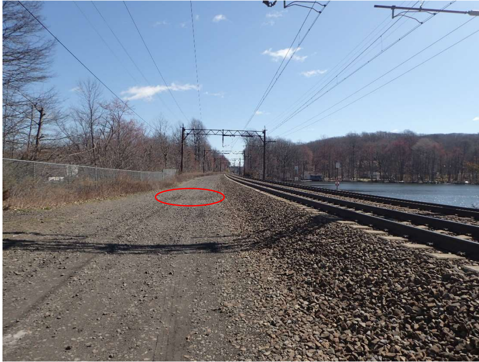
PHOTO 15: Concave surface on crest of dam looking northeast.
