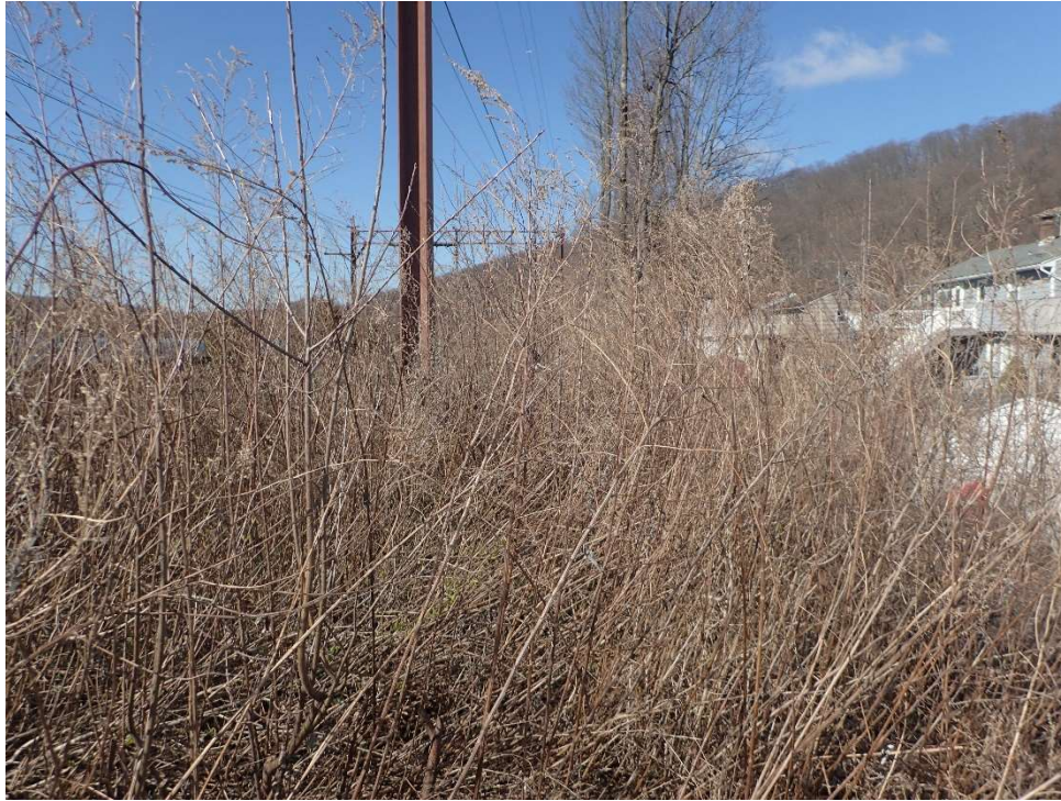
PHOTO 13: Previous area of clearing with excessive vegetation growth along downstream embankment looking southwest.
