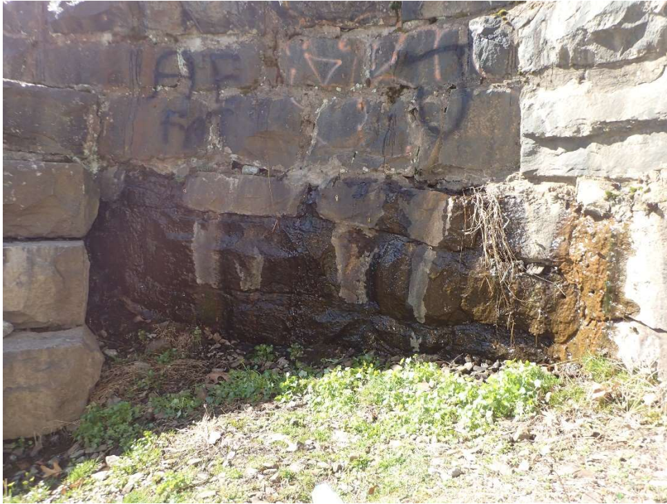
PHOTO 7: Joint deterioration and seepage at western spillway wingwall looking west.
